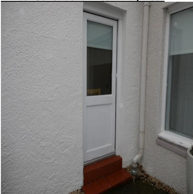
Timber Construction Rear Entry Door
