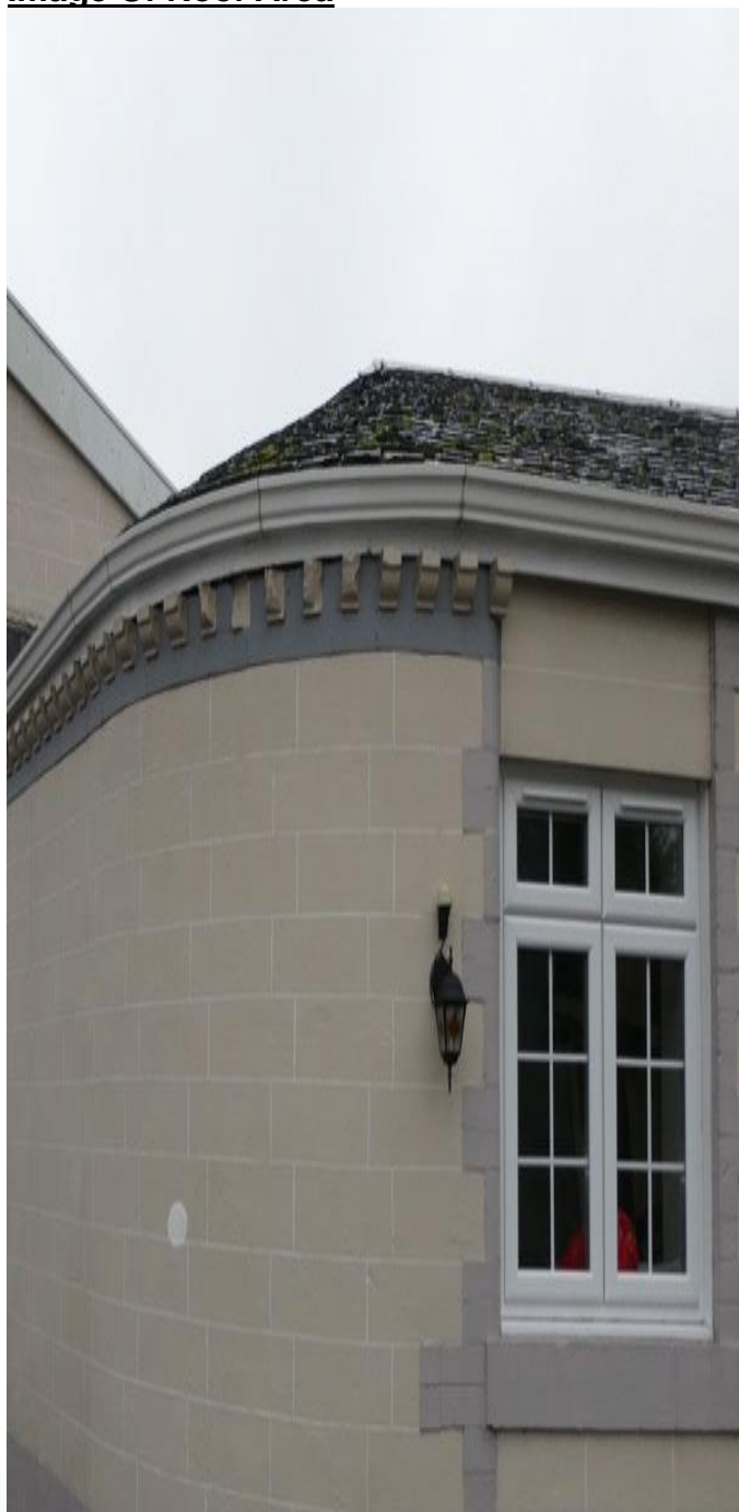
Image Of Roof Area
