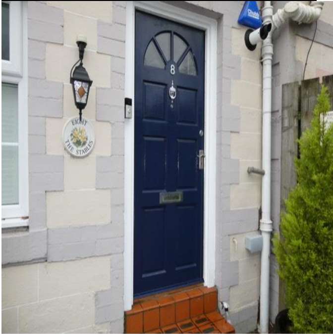
Timber Construction Front Entrance Door
