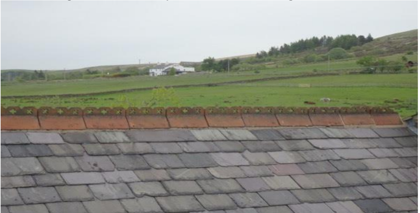
View of the ridge tiles to the central portion of the main building at the rear.
