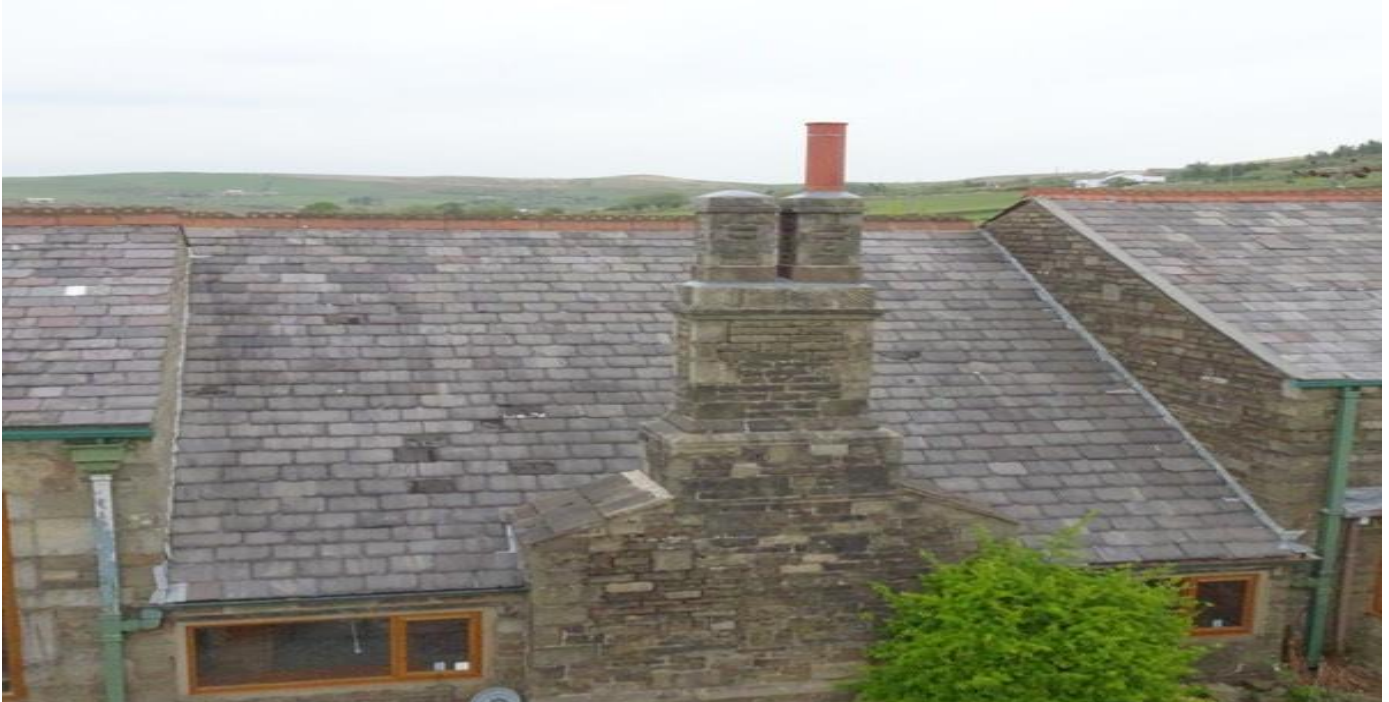
Overview of the roof and stone built chimney to the central portion of the main building at the rear.
