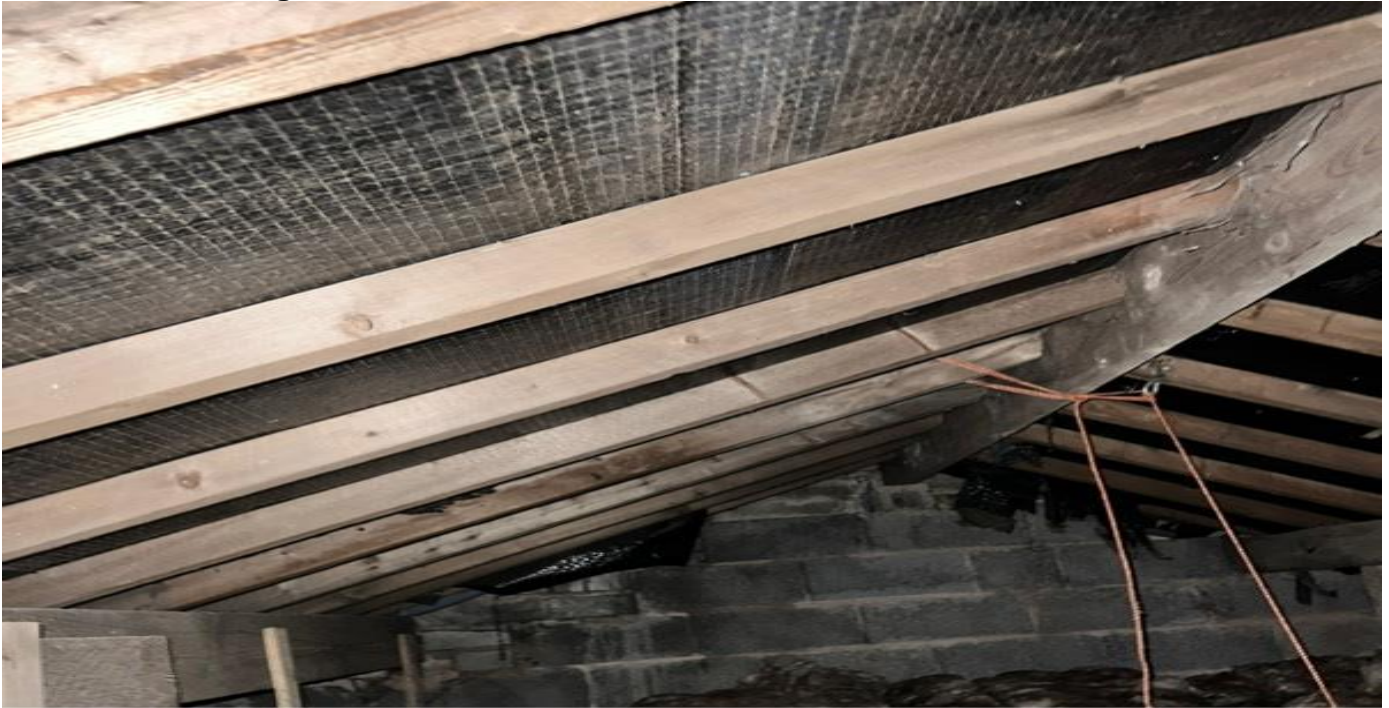
View of the sarking and internal timber roof structure.
