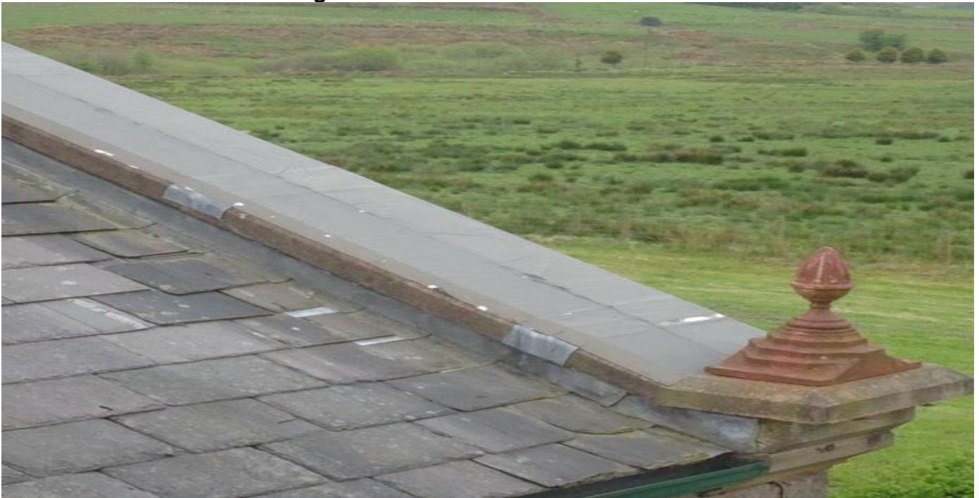
View of leaded abutments and the strip weather sealant to the stone coping at the right-hand side of the main building at the front.
