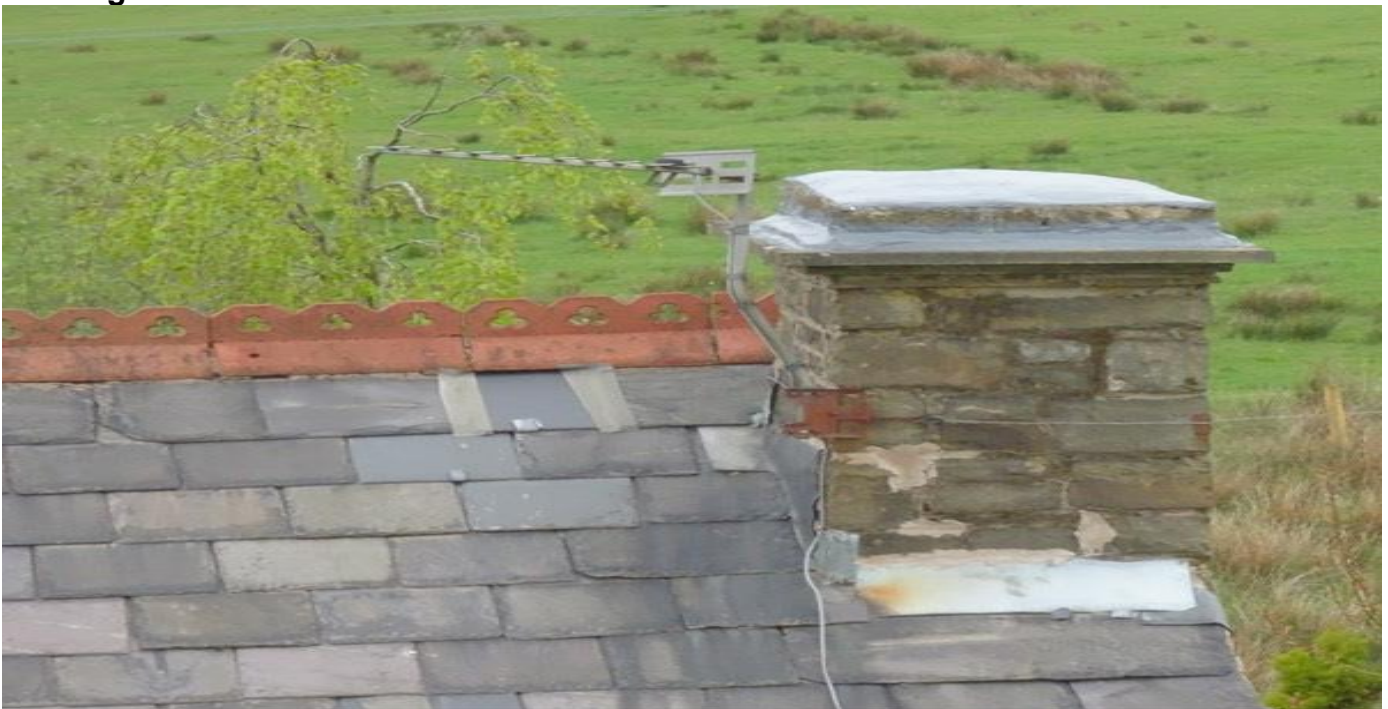
View of the redundant stone built chimney and ridge tiles to the right hand side of the main building from the rear.
