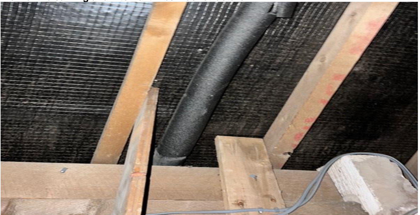
View of the sarking and internal timber roof structure.
