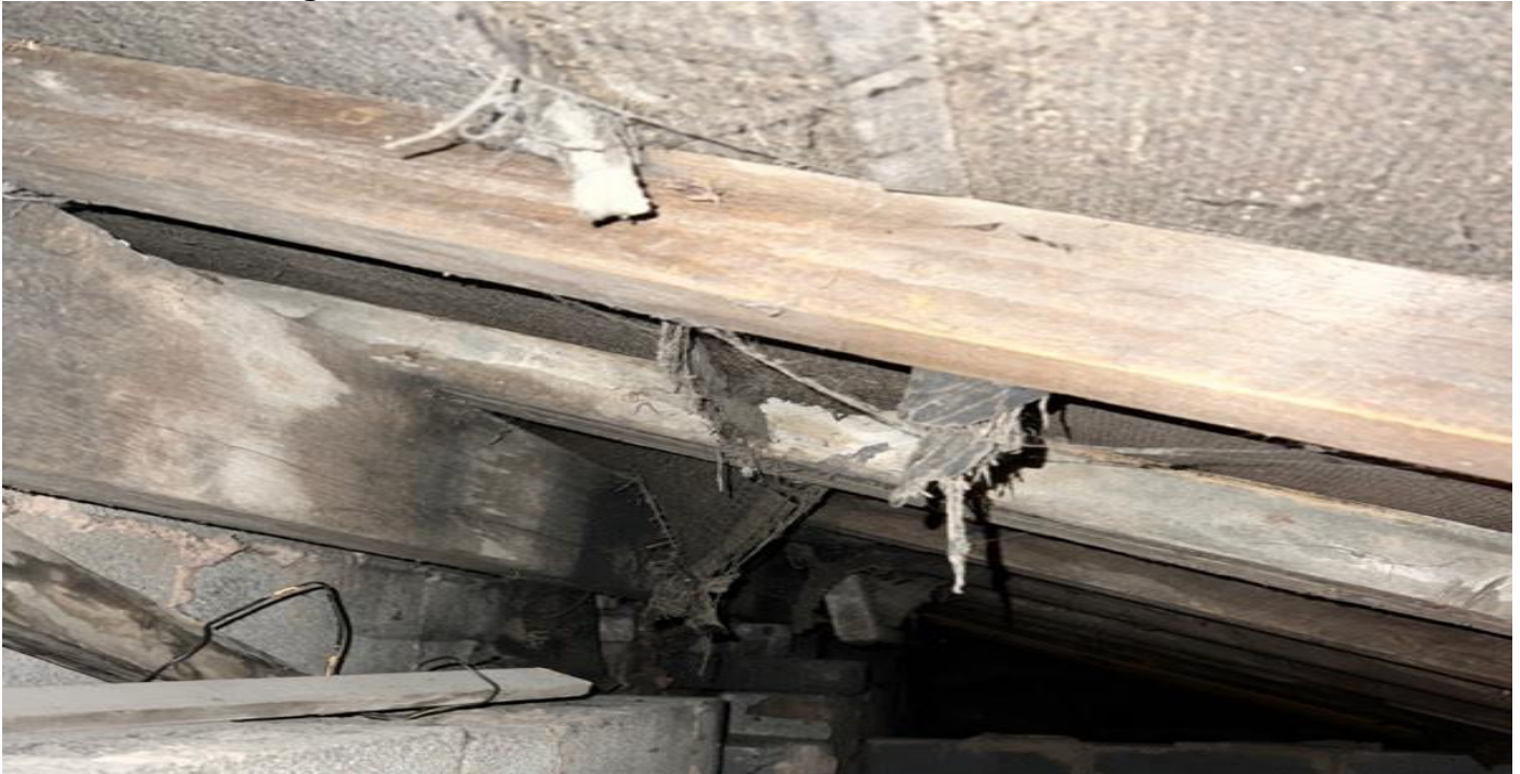
View of the sarking and rotting to the internal timber roof structure.
