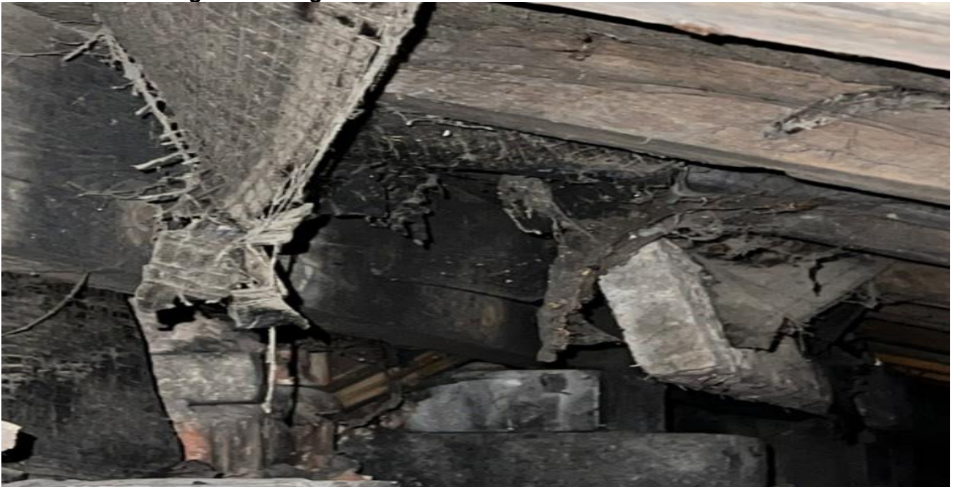
View of the sarking and rotting to the internal timber roof structure.
