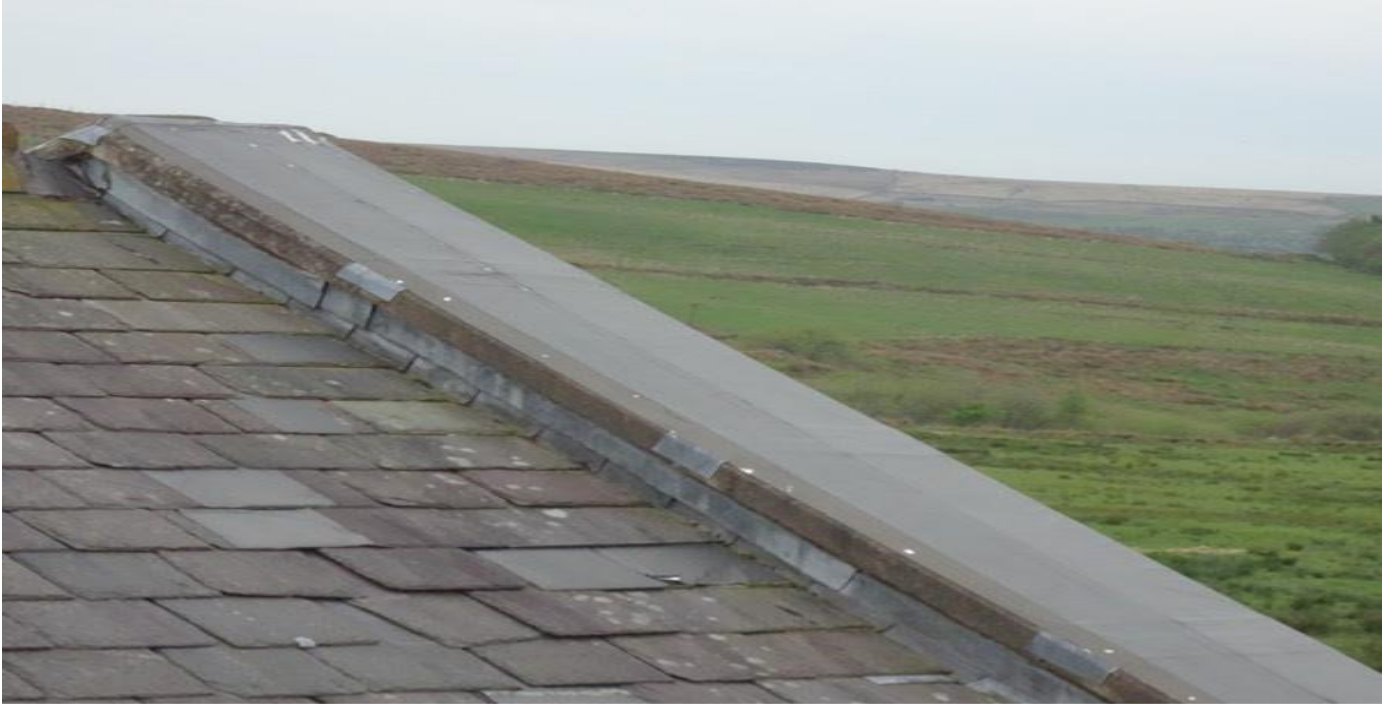
View of leaded abutments and the strip weather sealant to the stone coping at the right-hand side of the main building at the front.
