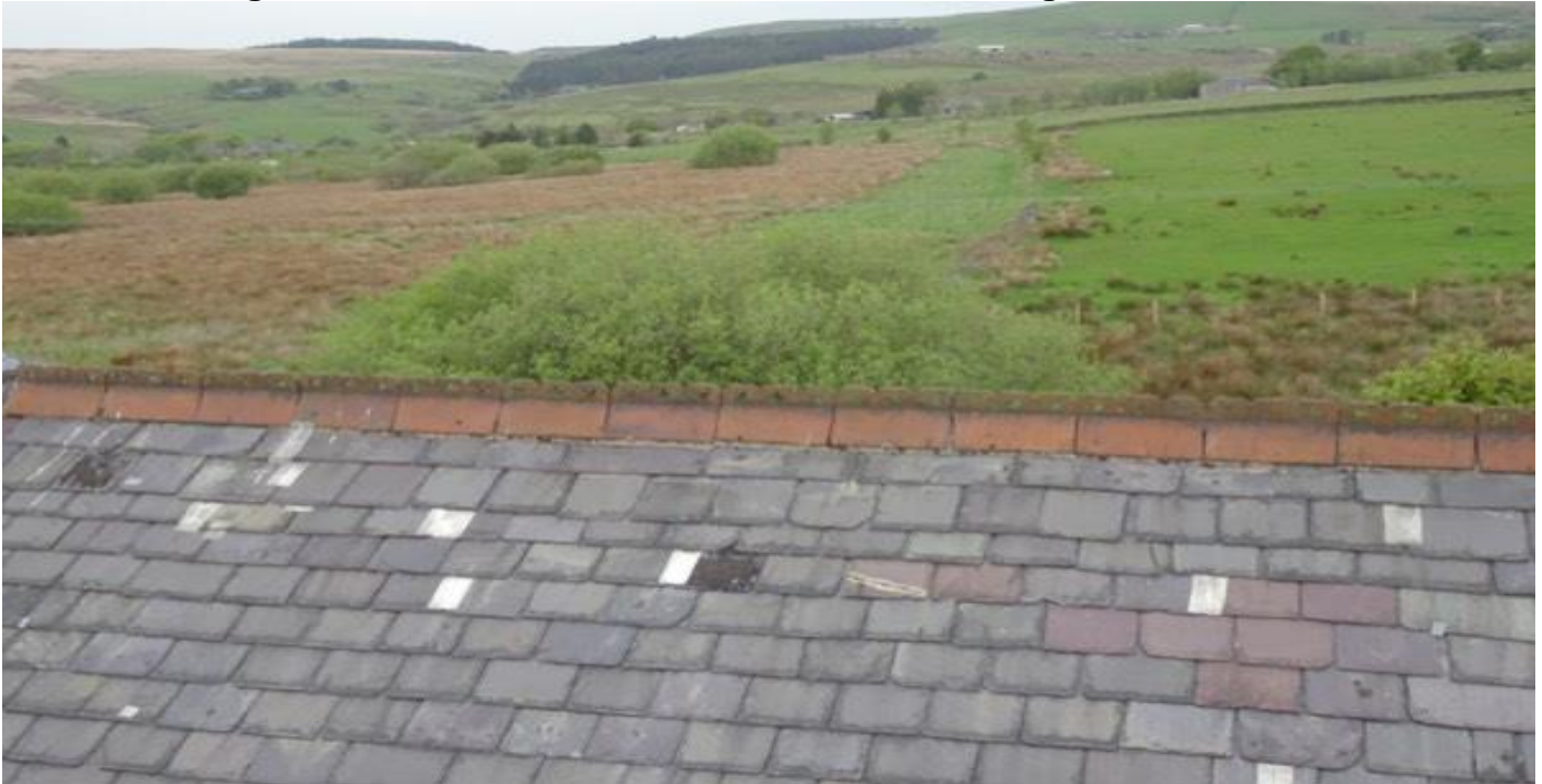
View of the ridge tiles, leaded abutments and coping to the left hand side of the main building from the rear.
