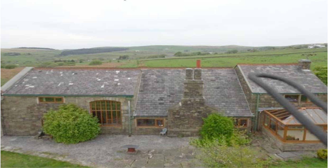
View of the redundant stone built chimney and ridge tiles to the right hand side of the main building from the rear.
