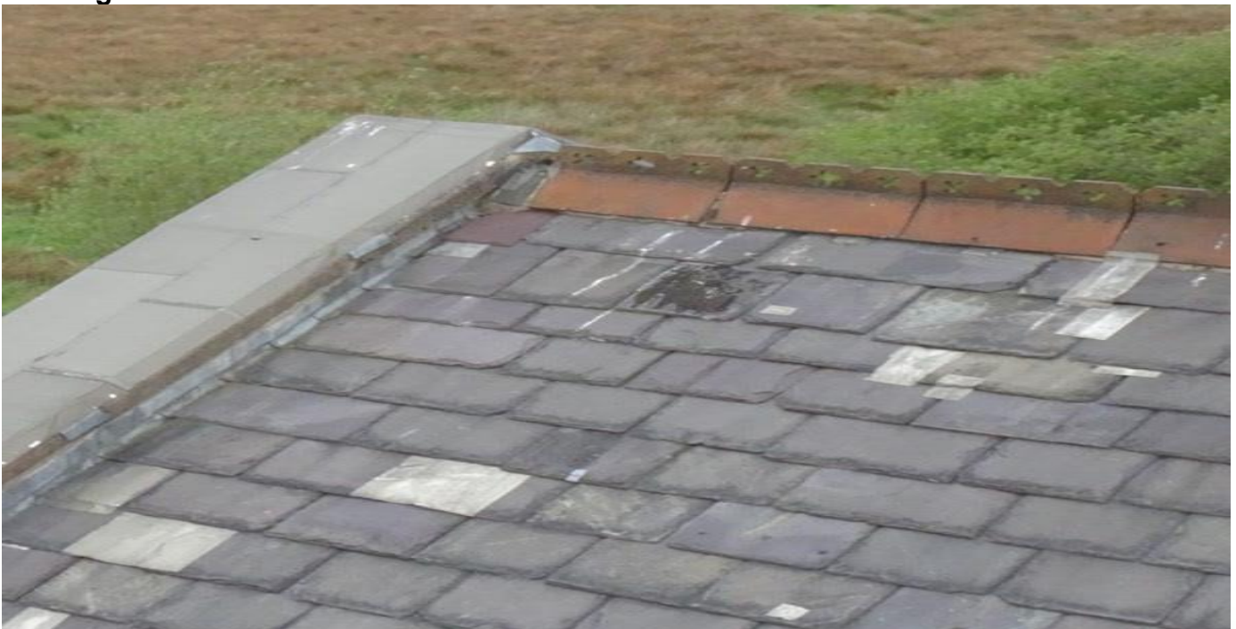
View of the ridge tiles, leaded abutments and coping to the left hand side of the main building from the rear.
