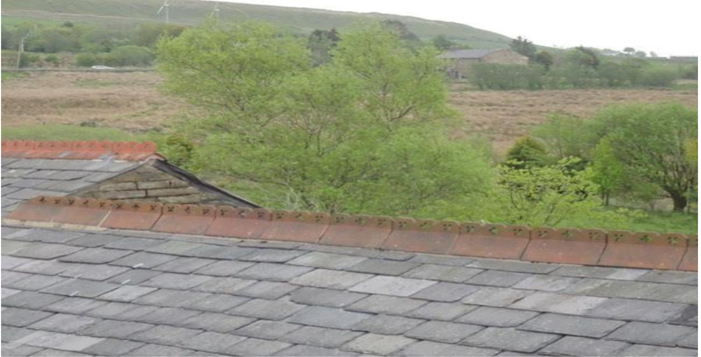
View of the ridge tiles to the central portion of the main building from the front.
