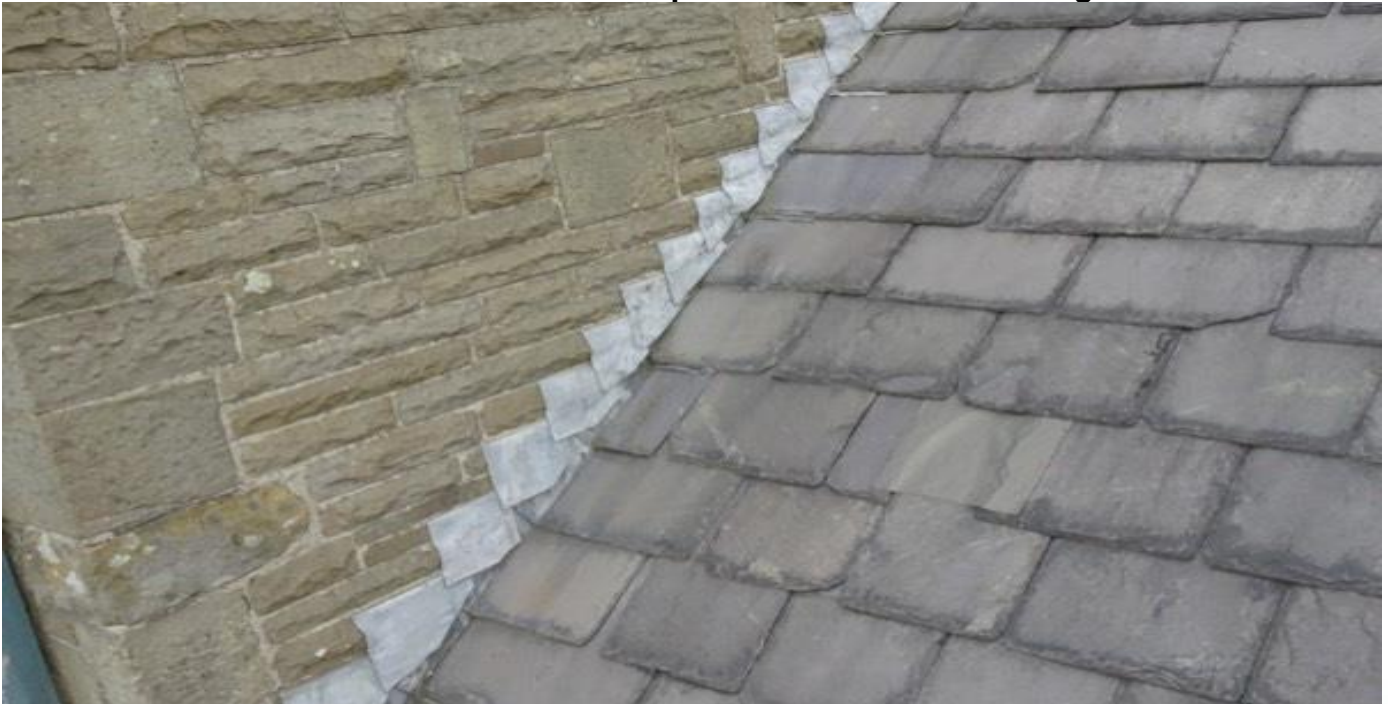
View of the leaded abutments to the central portion of the main building at the rear.
