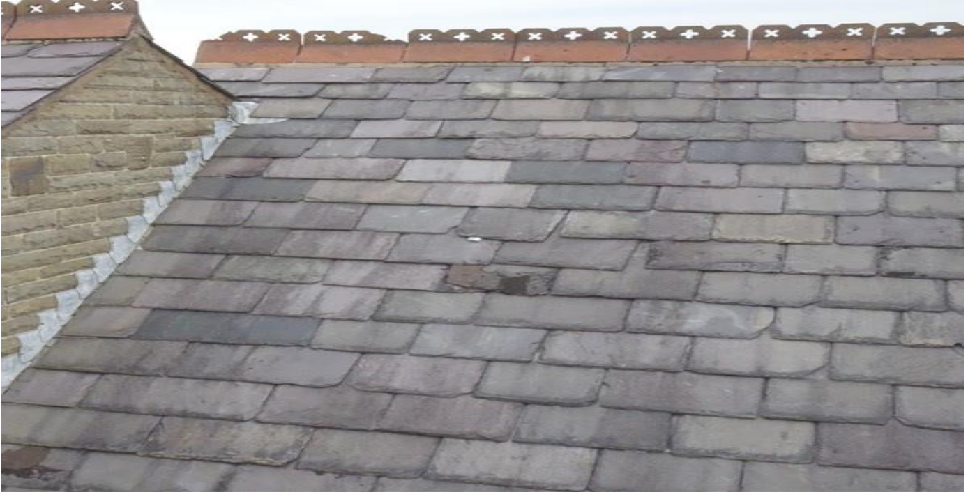
View of the leaded abutments to the central portion of the main building at the rear.
