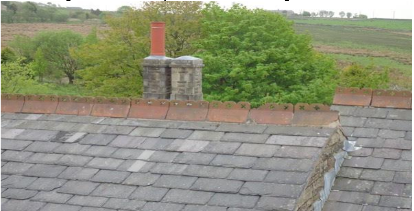
View of the ridge tiles to the central portion of the main building from the front.
