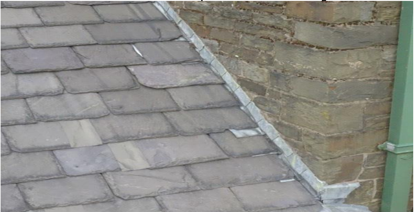
View of the leaded abutments to the central portion of the main building at the rear.
