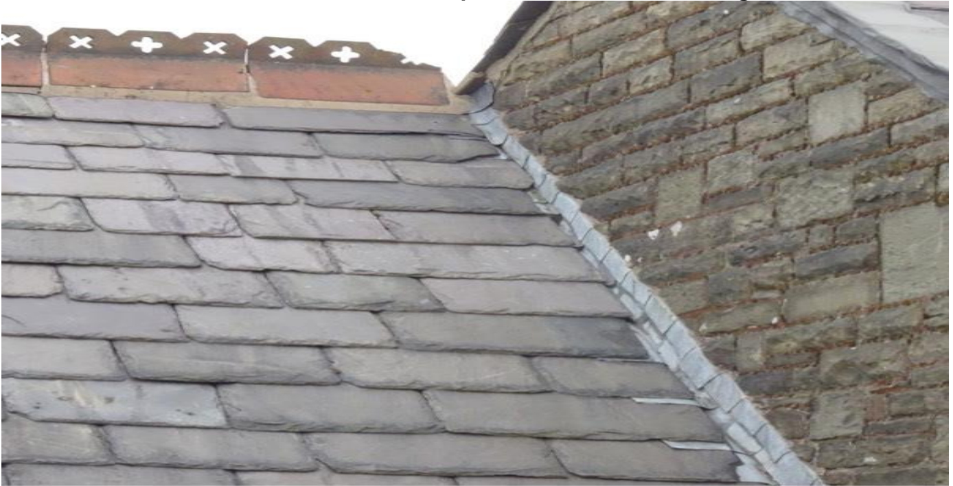
View of the leaded abutments to the central portion of the main building at the rear.
